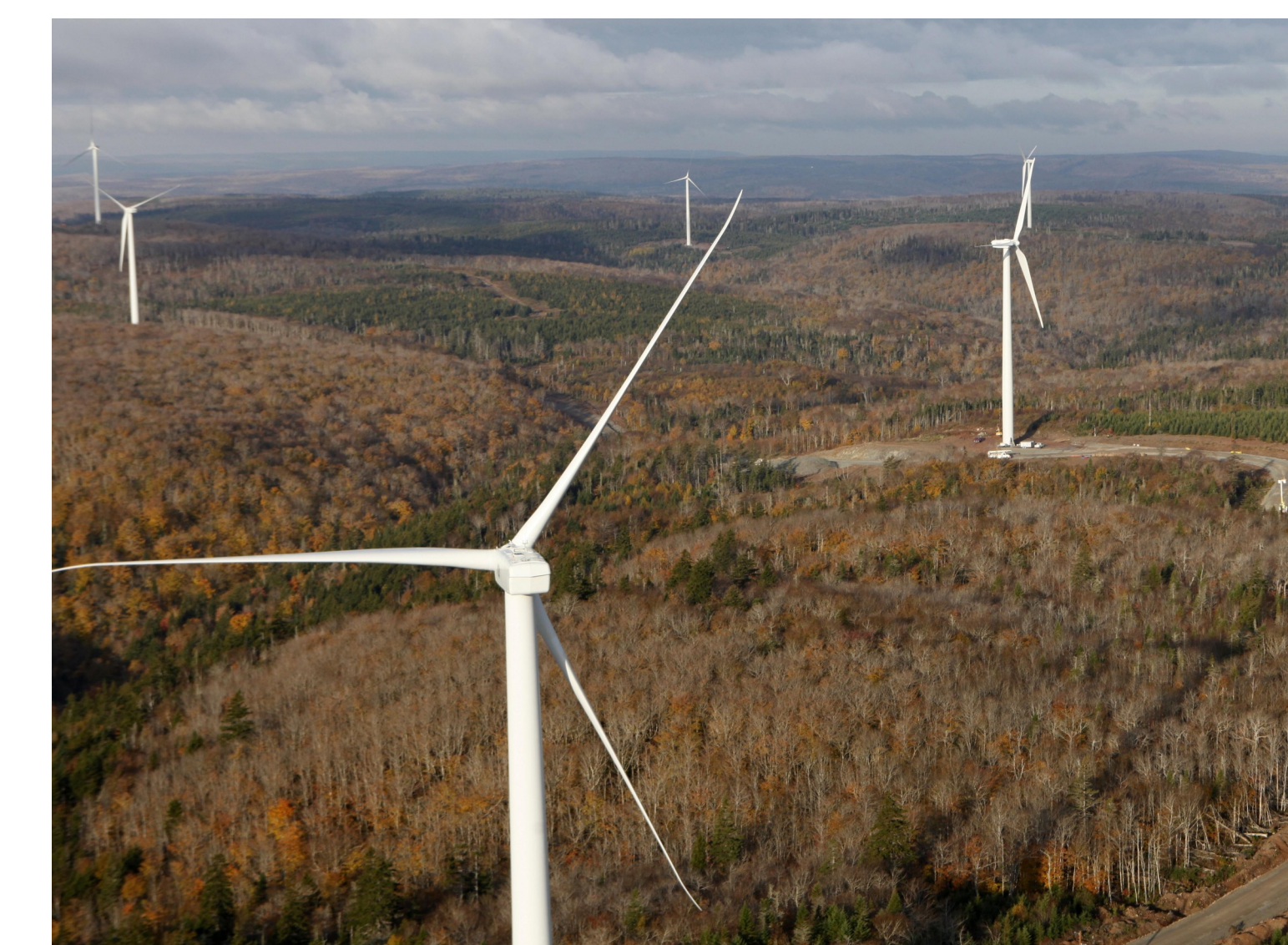
Dalhousie Mountain Wind Farm, Pictou County Image courtesy of Len Wagg, Communications Nova Scotia
